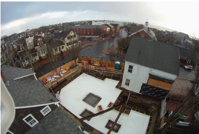
Foundation water-proofing
